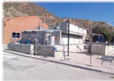
Anaerobic bioreactor (700 m 3 /day)
